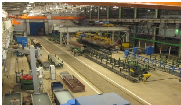
Figure 2 - A modern thermal zinc diffusion galvanising plant, capable of handling products up to 12 metres in length
